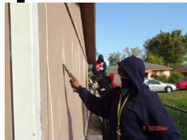
Southern University students prepping the wood siding for paint.
