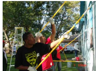
Volunteer students painting the south facade of the house.
